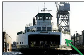
ALAN BERNER The 80-year-old Steel Electric-class ferry Quinault will not be returned to service unless the damage to its hull is repaired.
